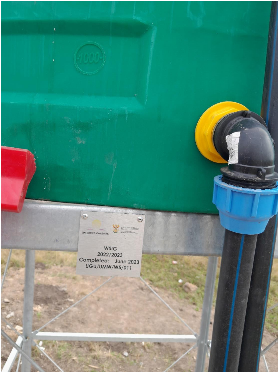
Fig 3 Borehole Reference Name Tag
