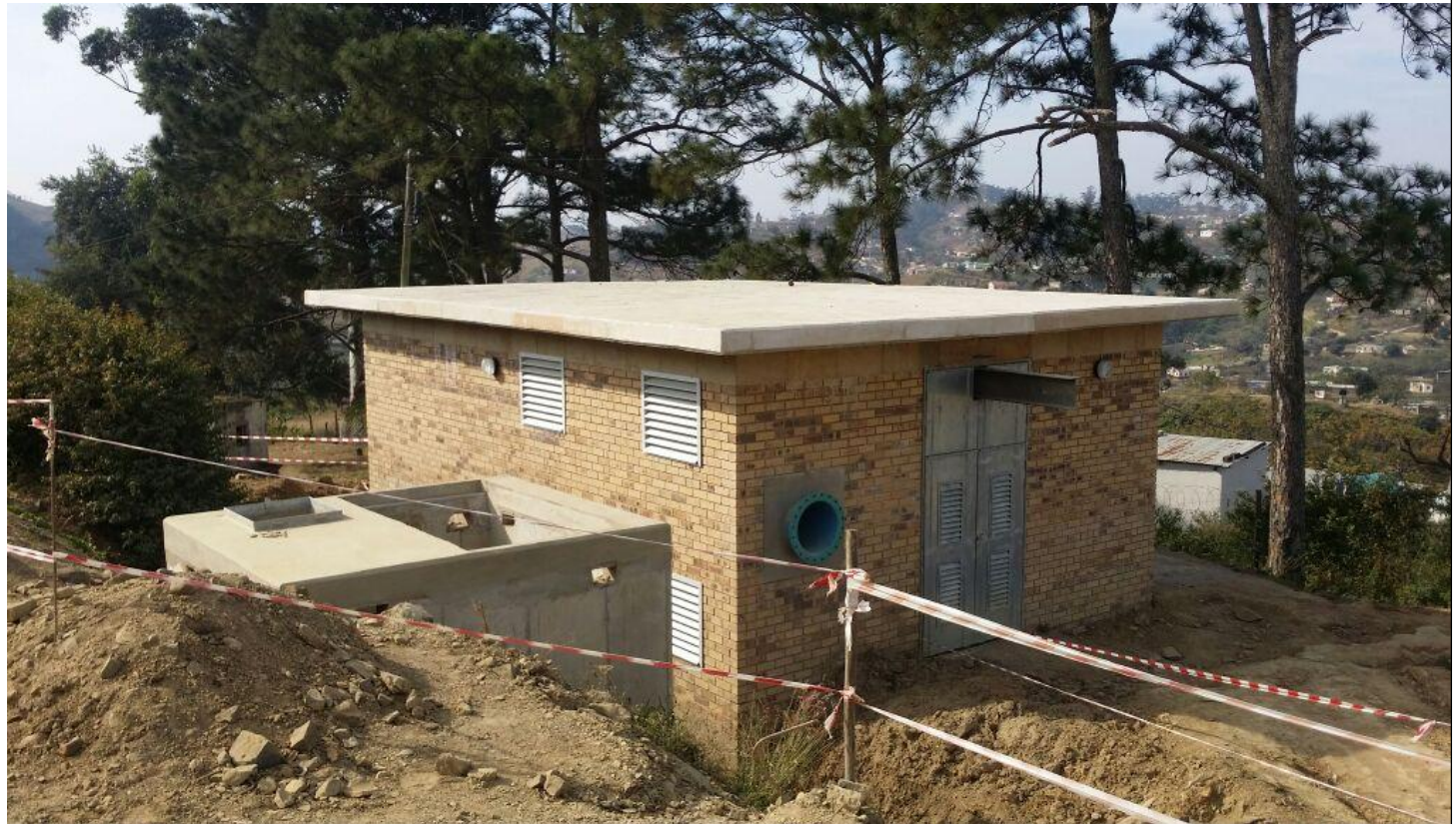
Treated Water pumpstation
