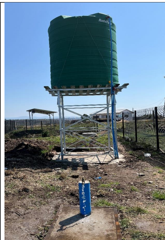
Completed Conversion of Handpump (Production Pump): KwaMachi Umuziwabantu Ward 05
