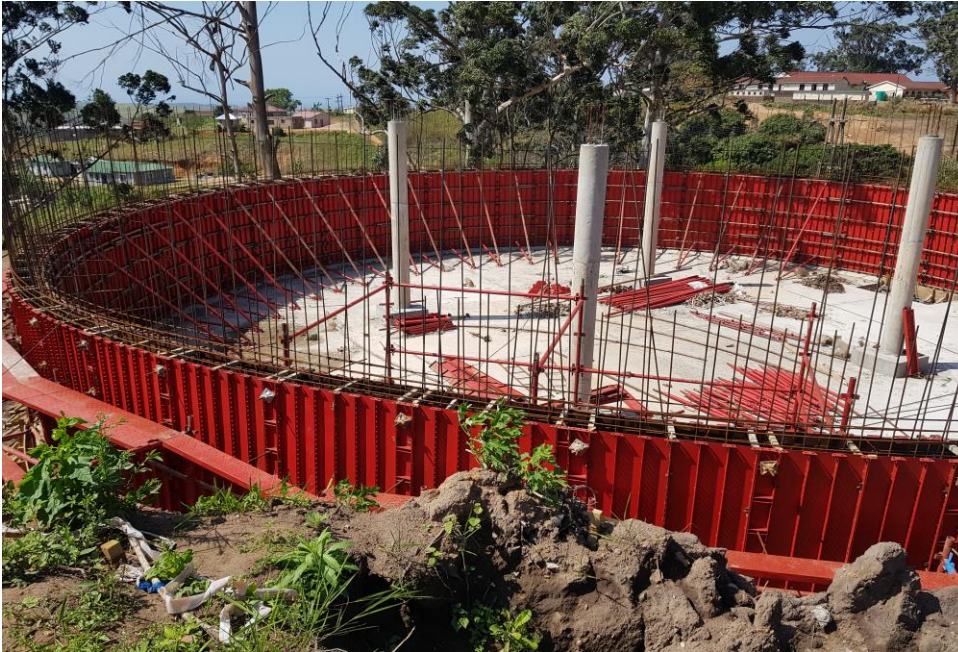
Construction of 2ML Reservoir
