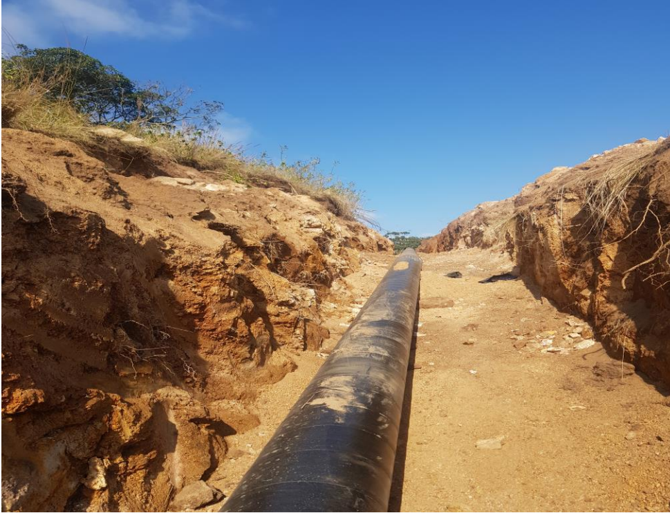
250mm Steel Pipeline Construction
