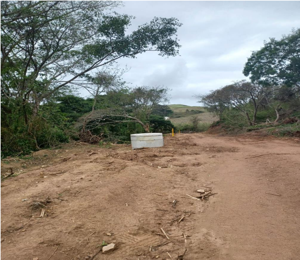
Complete 250mm Pipeline
