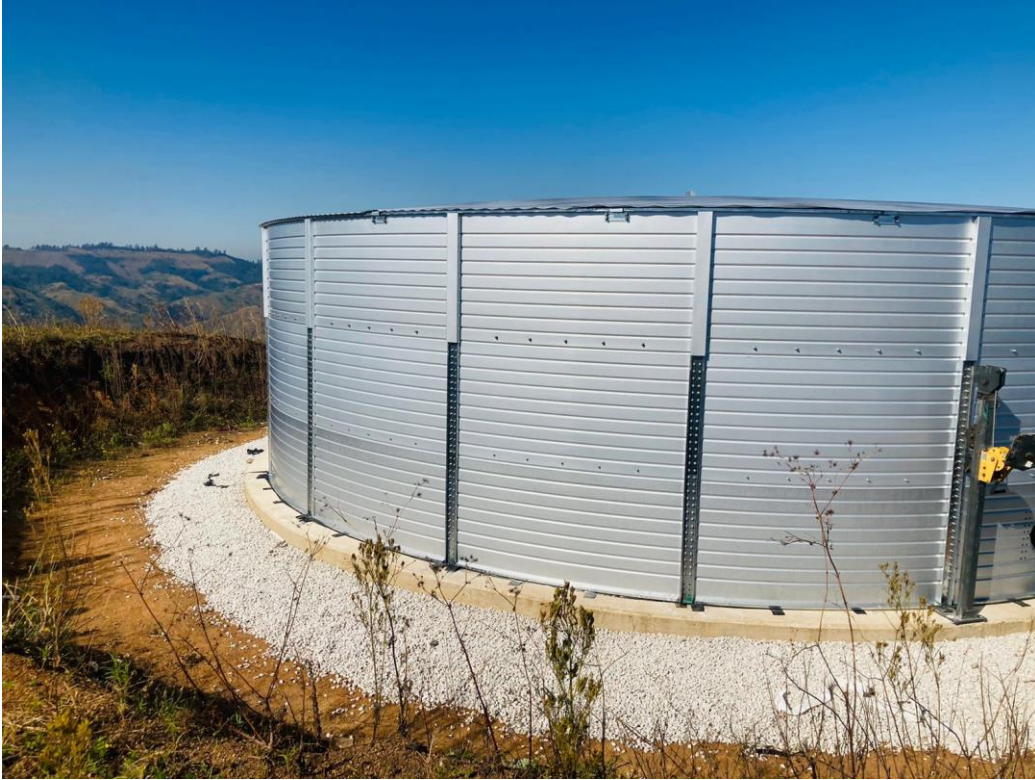
Construction of SBS Reservoir
