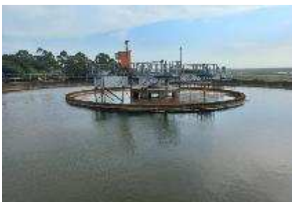
The clarifiers are generally in very good condition with very minimal floc carry- over
