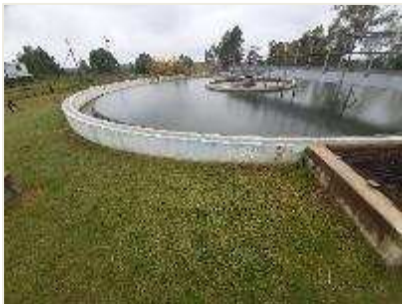
Sedimentation tank at Cullinan WTW
