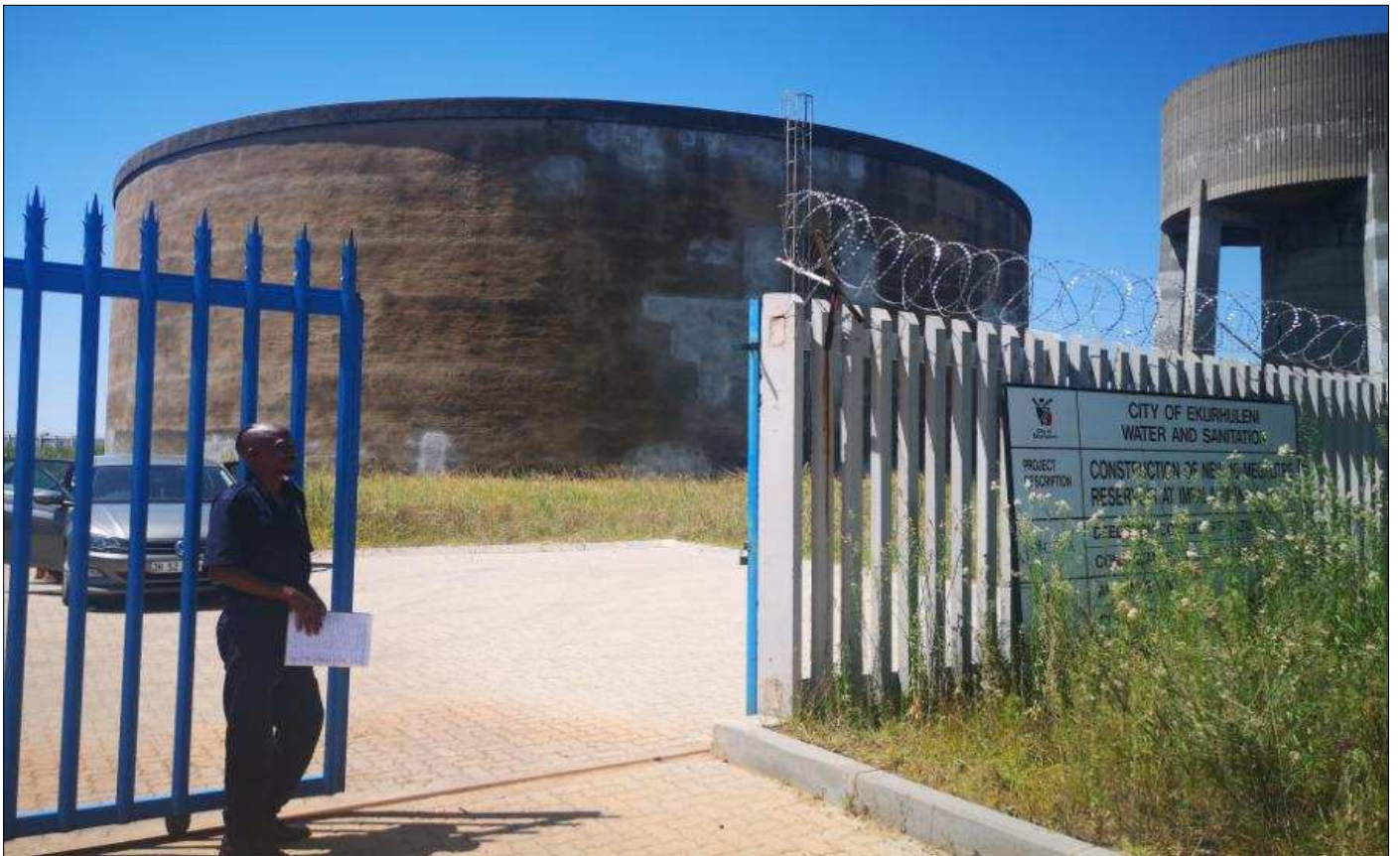
Impala reservoir secured, sign posted, neat terrain
