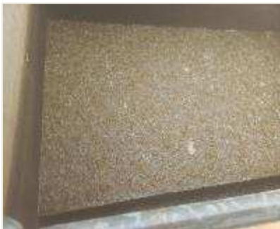
Filter backwashing at Cullinan WTW
