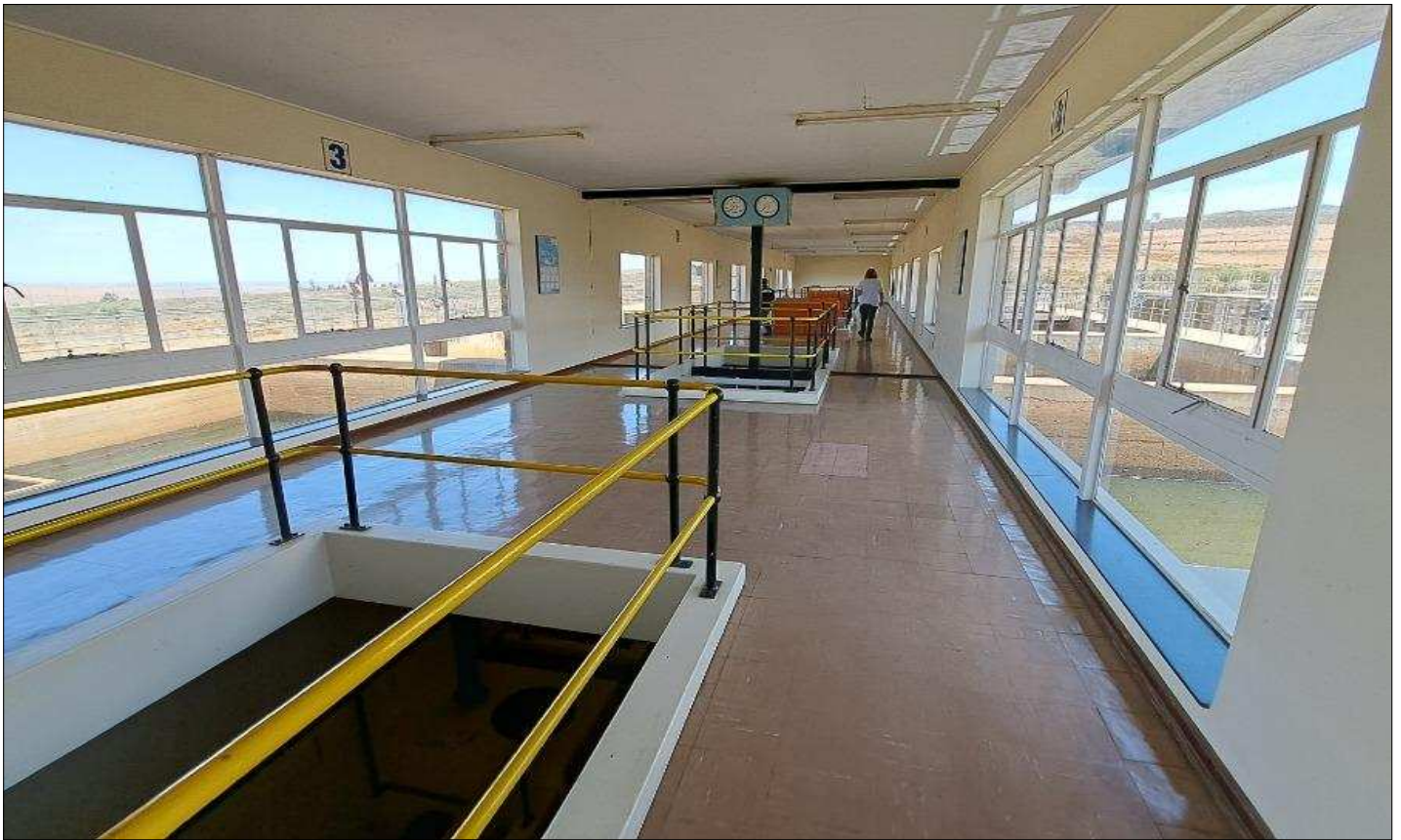
Saldanha Bay: Withoogte filter gallery – excellent operation and maintenance
