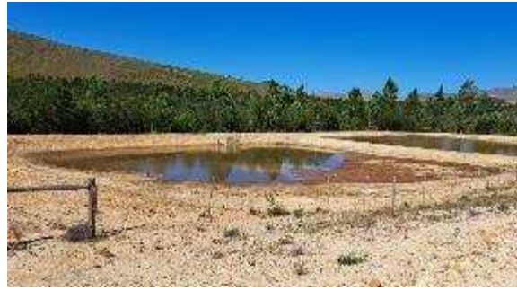
Sludge ponds at the Ruensveld West WTP
