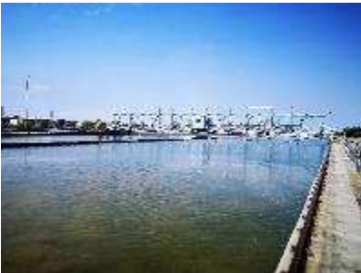
Sedimentation tank at Vereeniging
