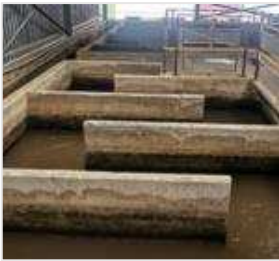
Flocculation Channel
