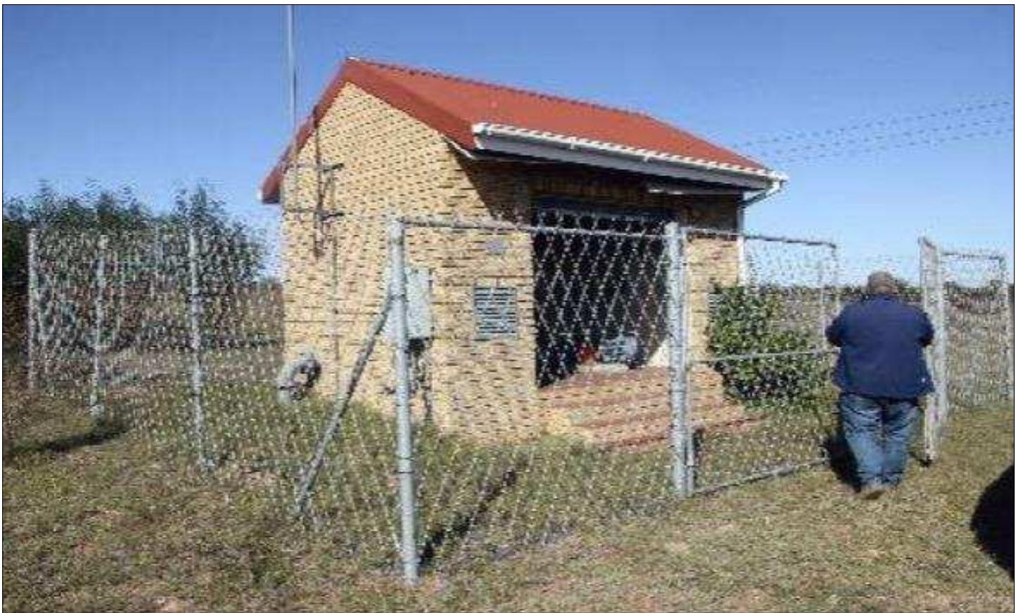
Swartland booster pumpstation and water network: Secured and well maintained
