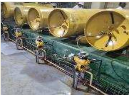
Chlorine storage tanks
