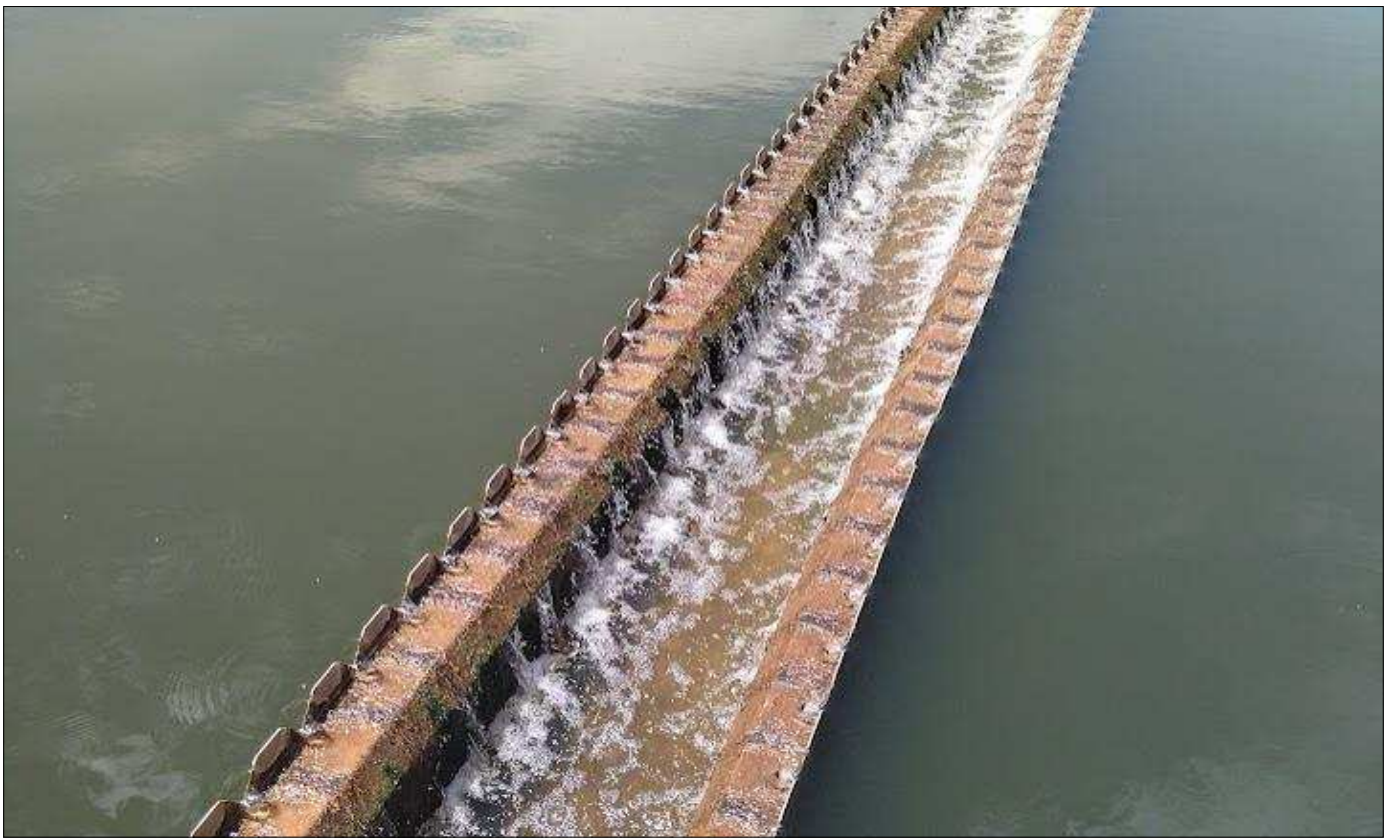
Withoogte clarification: Continuous strive to achieve SANS241 compliance
