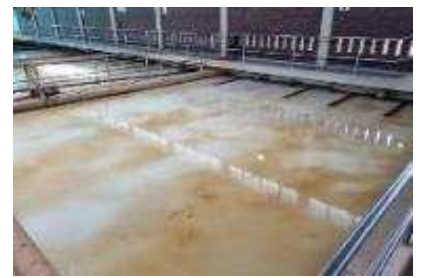
Excellent white-water and good DAF operation
