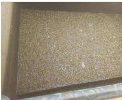
Filter backwashing at Cullinan WTW
