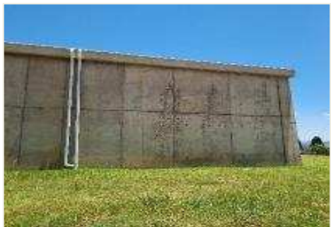
A well maintained bulk reservoir
