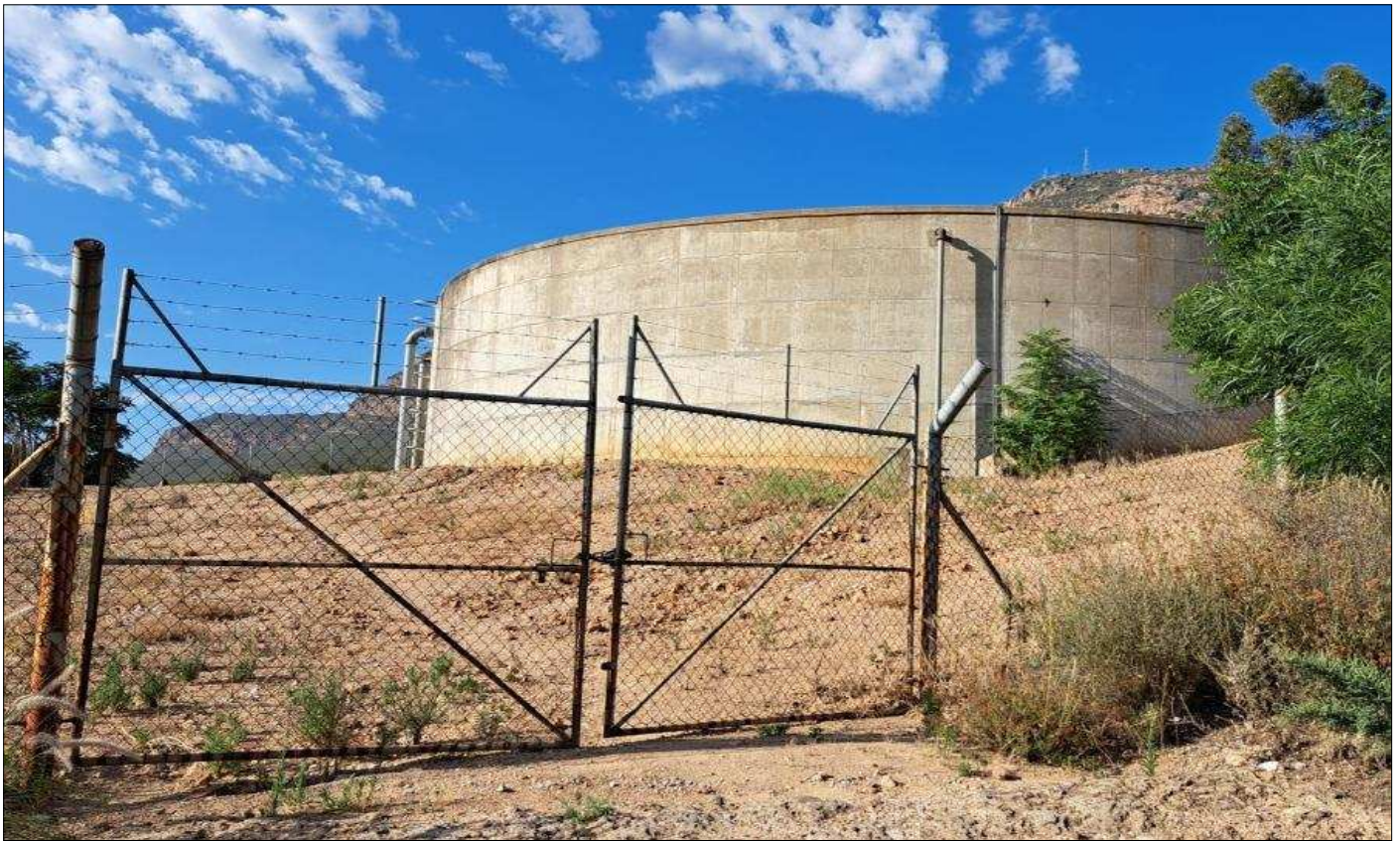
Piketberg reservoir secured with routine inspection regime
