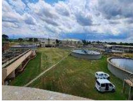
The plant surrounding is well maintained
