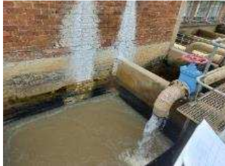
Flow splitting to module 1 and 2
