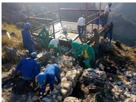
Figure 3 : View Deck pergola railings being installed and completion of walkway leading to the first view deck.
